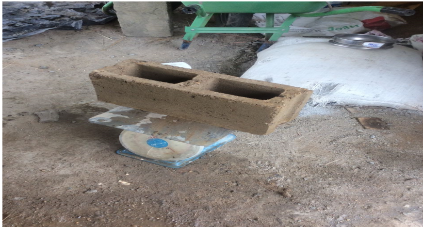
Figure 3.3 - Weighing of 6-inch hollow sandcrete block.
