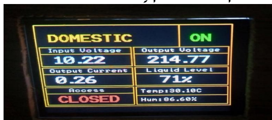
Fig. 6: TFT LCD Screen Result Showing Transformer Parameter
