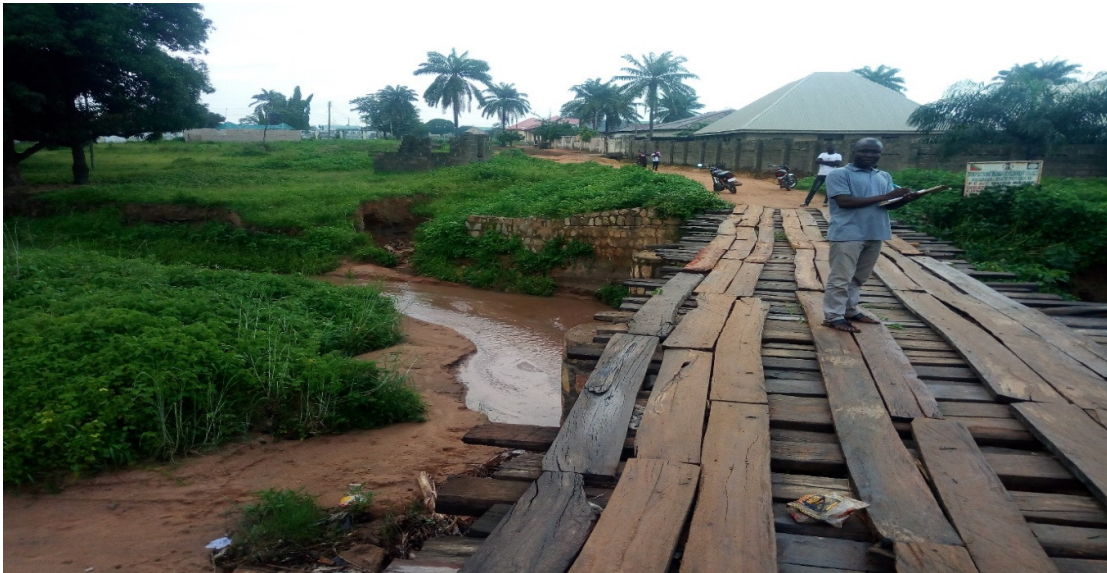
Plate 8: A typical gully cross-section in Farinruwa, Wamba LGA Source: Field work.
