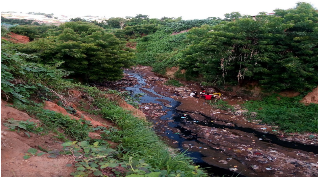
Plate 4: A typical gully cross-section in Tudun-Allu, Lafia LGA Source: Field work.
