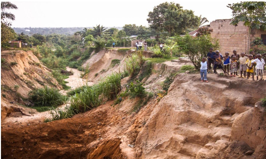
Plate 3: Linear shaped gully in Kwandere site, Lafia, LGA Source: Field work.
