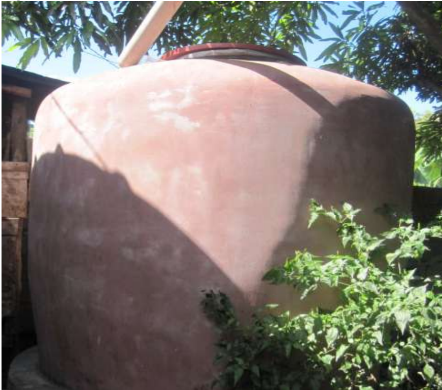
Fig. 3.28: A finished Rainwater Harvesting Tank
