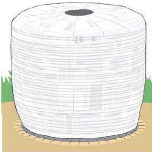
Fig. 3.13: Winding some wire around the tank to hold the paper
