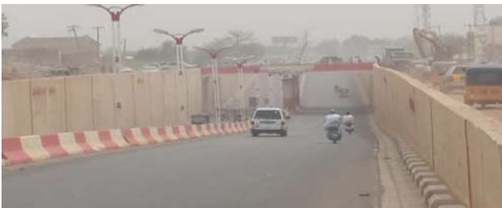
KofarGadon Gaya (Prince Abubakar Audu) Underpass Bridge
