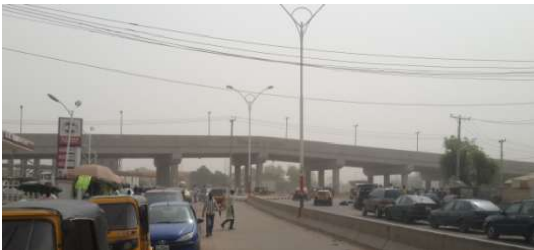
Ado Bayero (GadarLado) Flyover Bridge, Zaria Road
