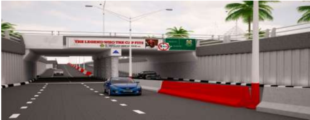
Panshekara/Madobi Junction Underpass Bridge(Under construction)
