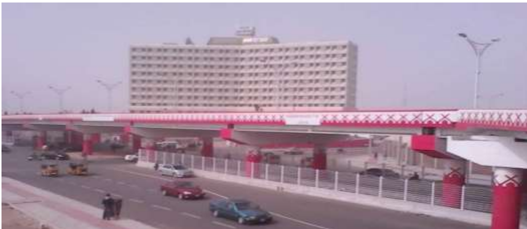
Ibrahim Taiwo (Olusegun Obasanjo) Flyover Bridge
