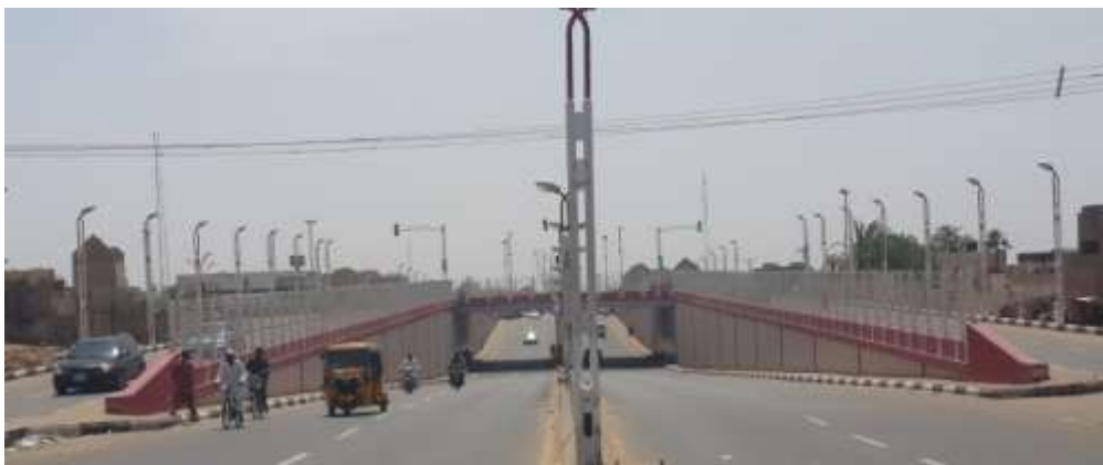
KofarKabuga (General Ibrahim Badamasi Babangida) Underpass Bridge
