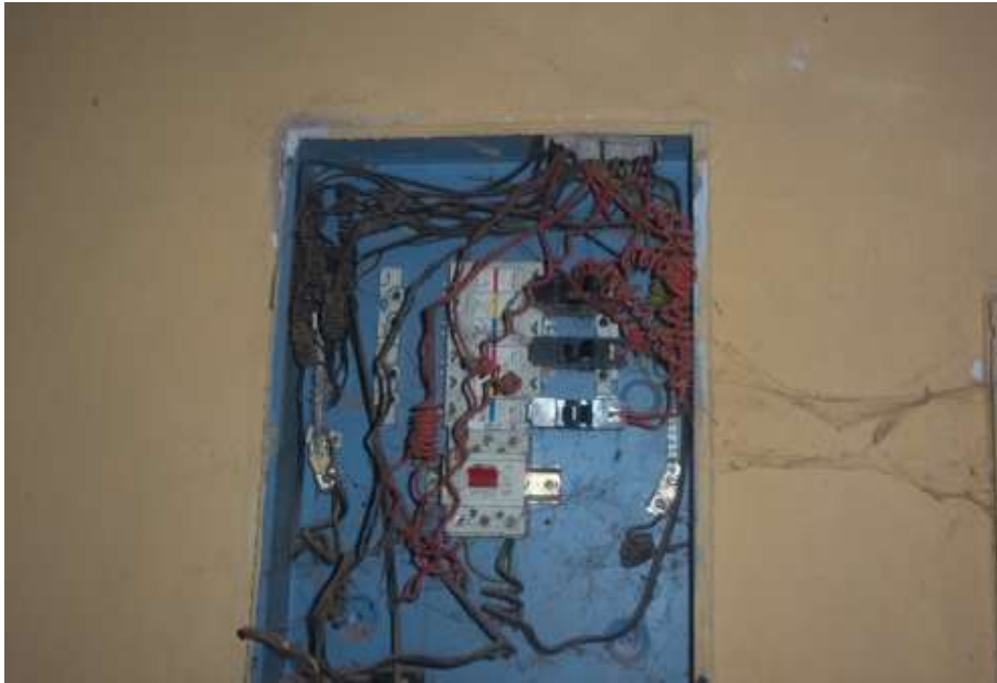
Fig 2: By-passed distribution board
