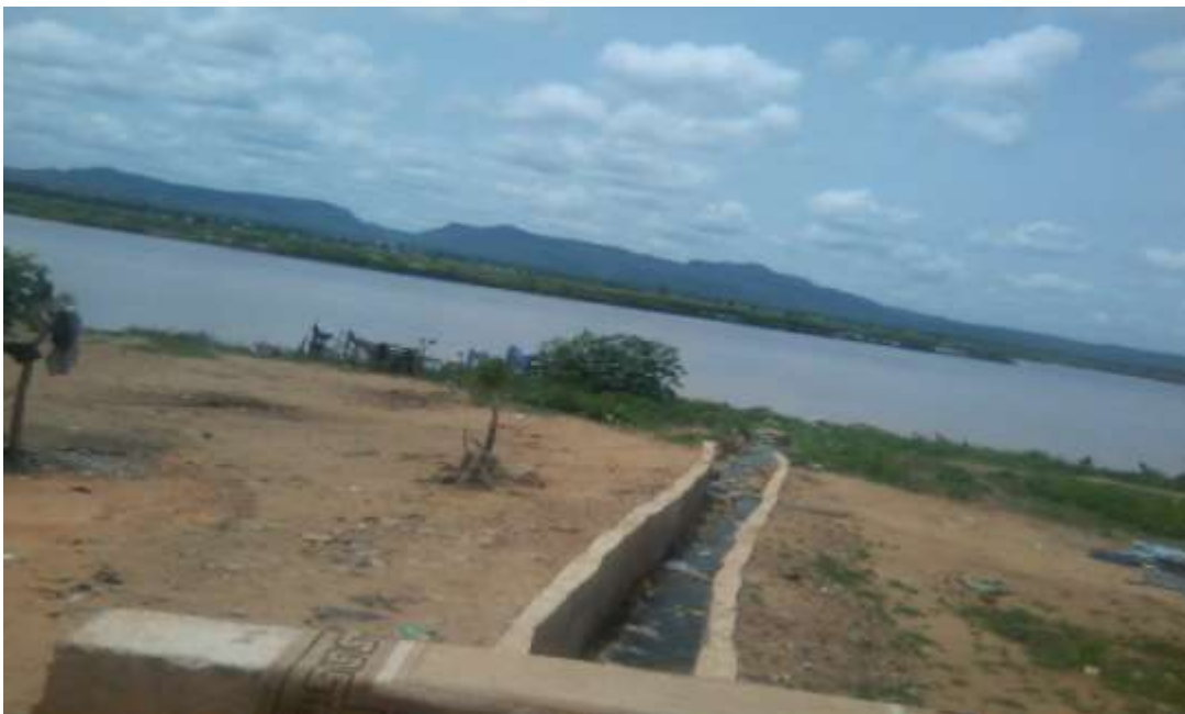
Figure 4.7: Blockage drainage that goes through River Benue
