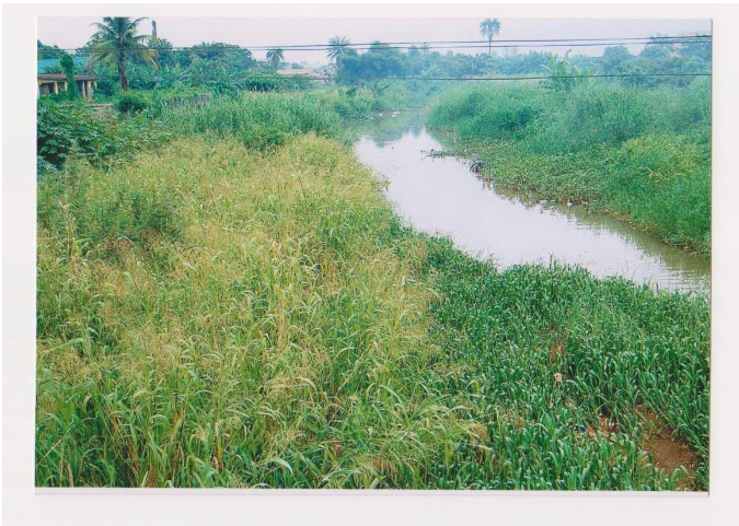
Figure 1:- Narrowed Channel as a Result of Vegetation cover Source (Author).
