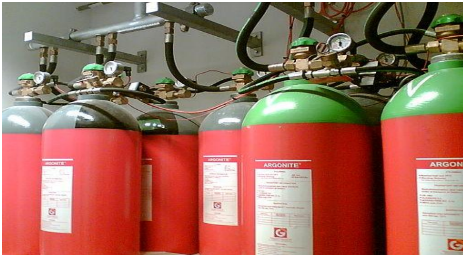
Plate II: Automatic Fire Suppression System [Source: Word Press, 2013 ( https://bestfiresuppressionsystems.wordpress.com/ )].
