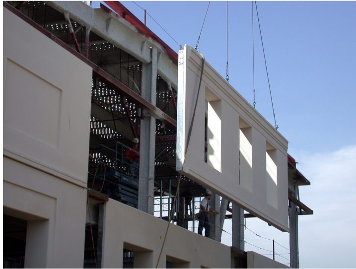
Figure3: Showing Modular Sections
