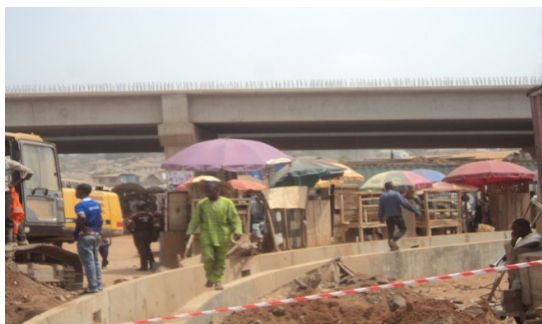
Plate 3: The Sapon fly over under construction.
