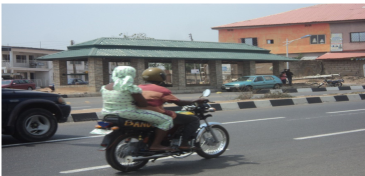
Plate 6: Modern bus stops along Ibara – Sokori – Totoro road Source: Authors' field work, 2014
