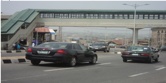
Plate 5: Modern pedestrian bridge on Ibara – Sokori – Totoroad Source: Authors' field work, 2014
