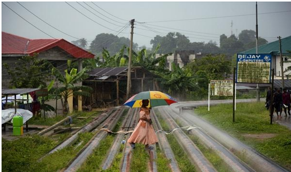
Figure 2: Erosion exposes Oil pipelines in a community of Okrika. Source: Circles of Blue, 2009.
