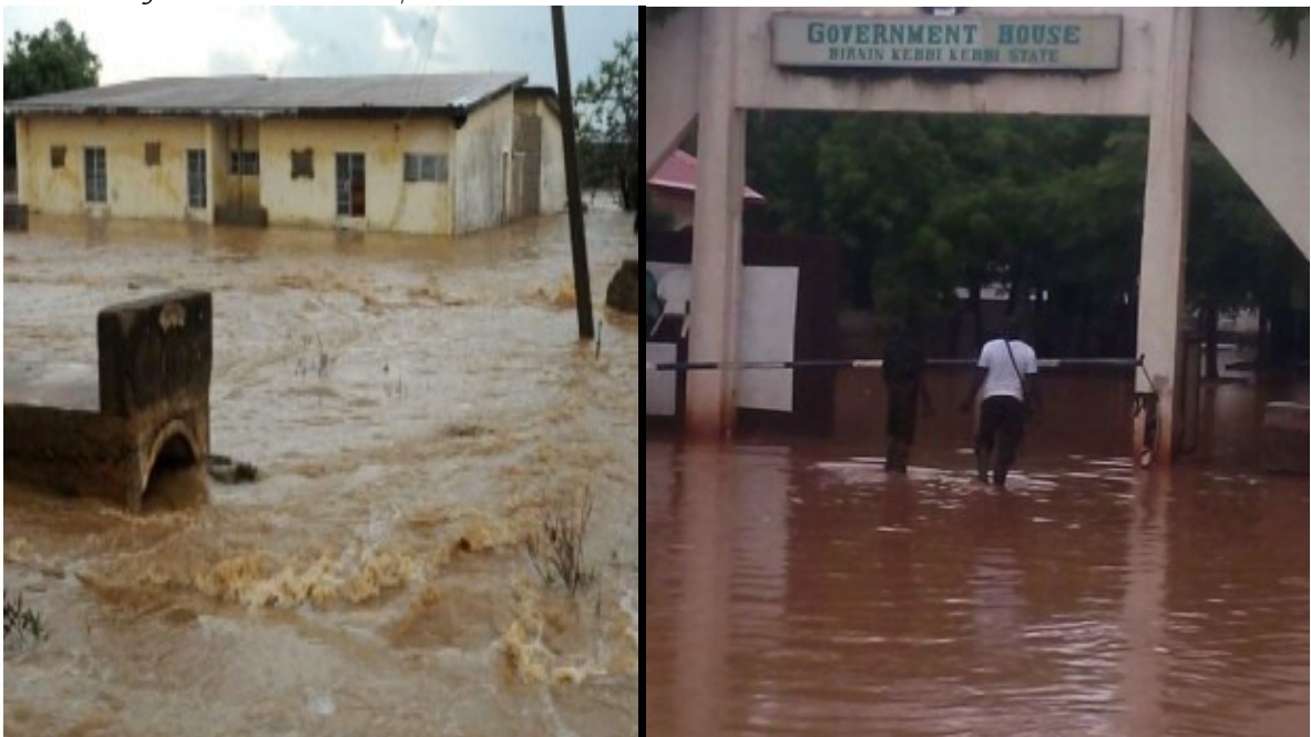
Plates 1.2 showing 2014 flooding in Bayan Kara Residential area and Government house in Birnin Kebbi.
