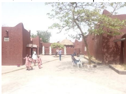
Plate III: Museum gallery buildings showing the dark red colour consistent on the buildings
