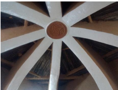
Plate X: One among the various arch composition of Hausa architecture serving as ceiling to the interior
