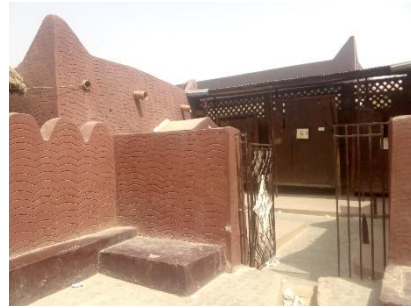
Plate II: A section of the museum showing the various vernacular features described
