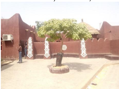
Plate VIII: Motifs on buttresses that breaks the monotony of the vast horizontal stretched walls
