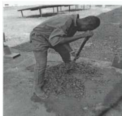
Fig. 3.3: Concrete Mixing
